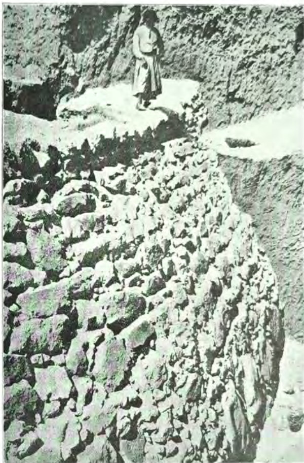
FIG. 90.—Foundation of the city-wall of Jericho. (By permission from the Mitteil. d. Deutsch. Orient-Gesellschaft (No. 39, abb. 7.)
