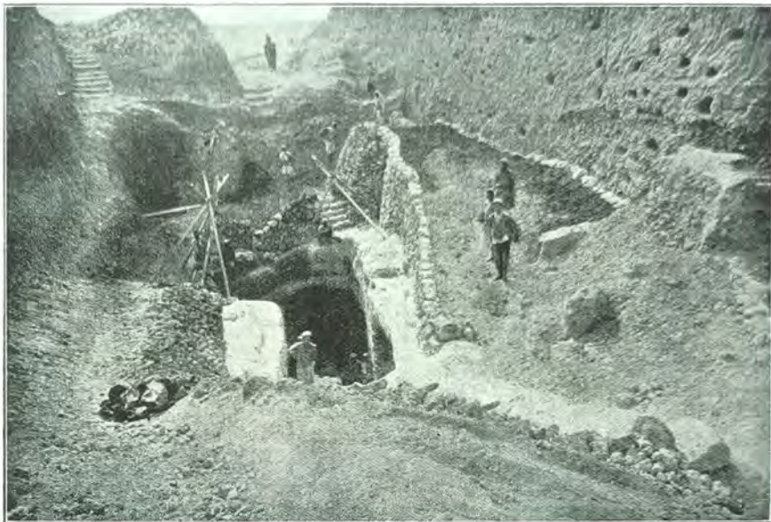
FIG. 85.—The Entrance to the Tunnel (from the north).
