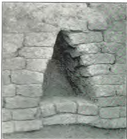
Corbelled Arch of Crude Bricks About 2500 B. C.
