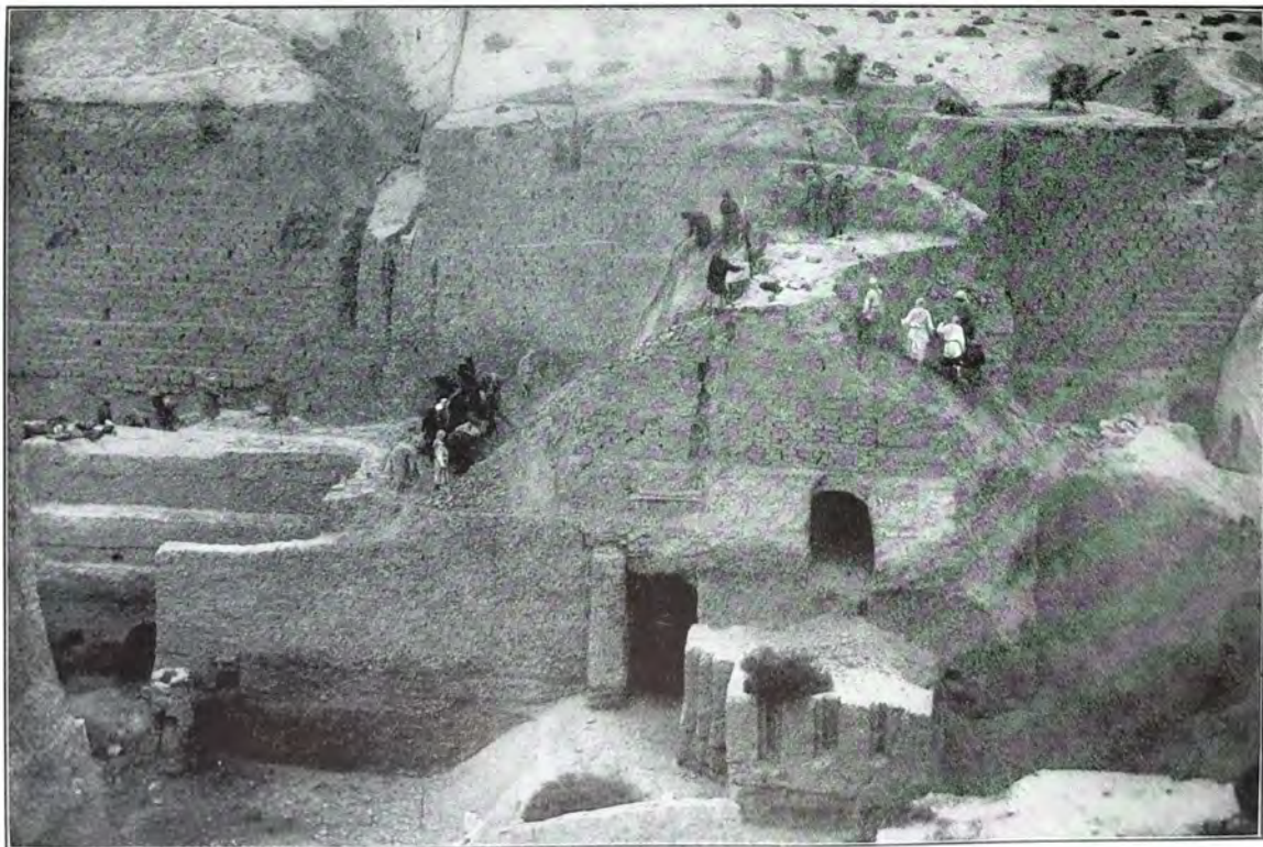
The Removal of a Tower of the Seleucido-Parthian Fortress and the Clearing of the Ancient Temple Gate beneath it
