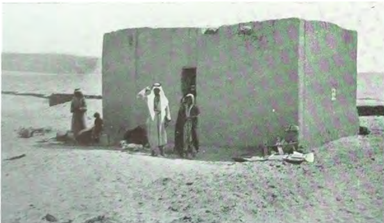
Fig. 55. Modern mud-brick house near Ezion-geber, its wall not bonded together as in the case of its ancient prototype.
