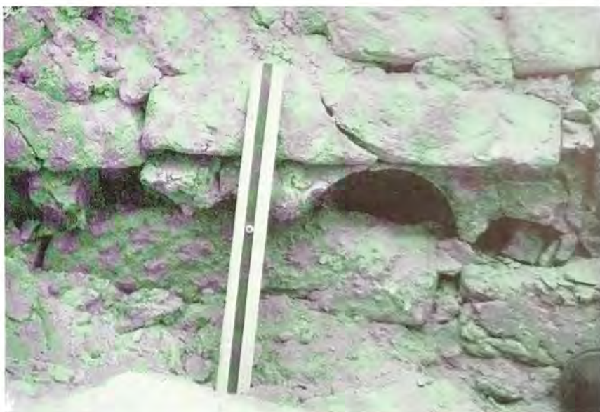
Fig. 48. Flues in the south wall of furnace room 1 in the refinery at Tell Kheleifeh.
